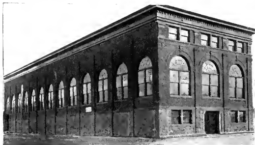
FIG. 2.—DOCK STREET SUB-STATION, SCHENECTADY.
